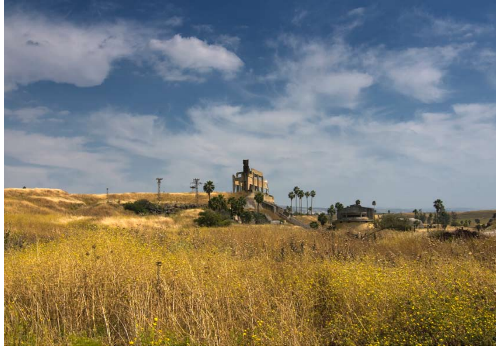
View of the hydroelectric power station from the Peace Island.
