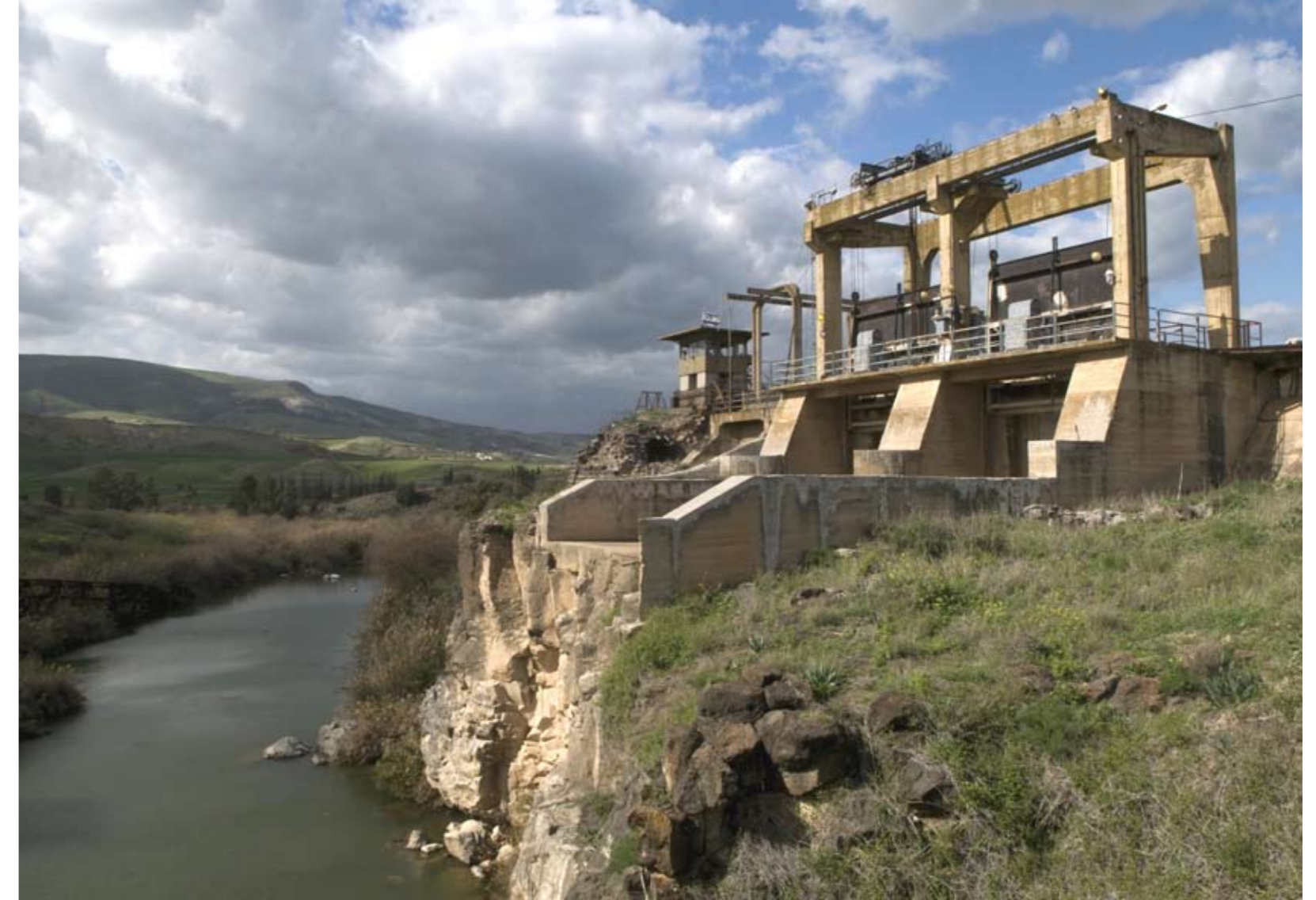
The architecture of the power station is striking in its bold, streamlined, modernist forms.
