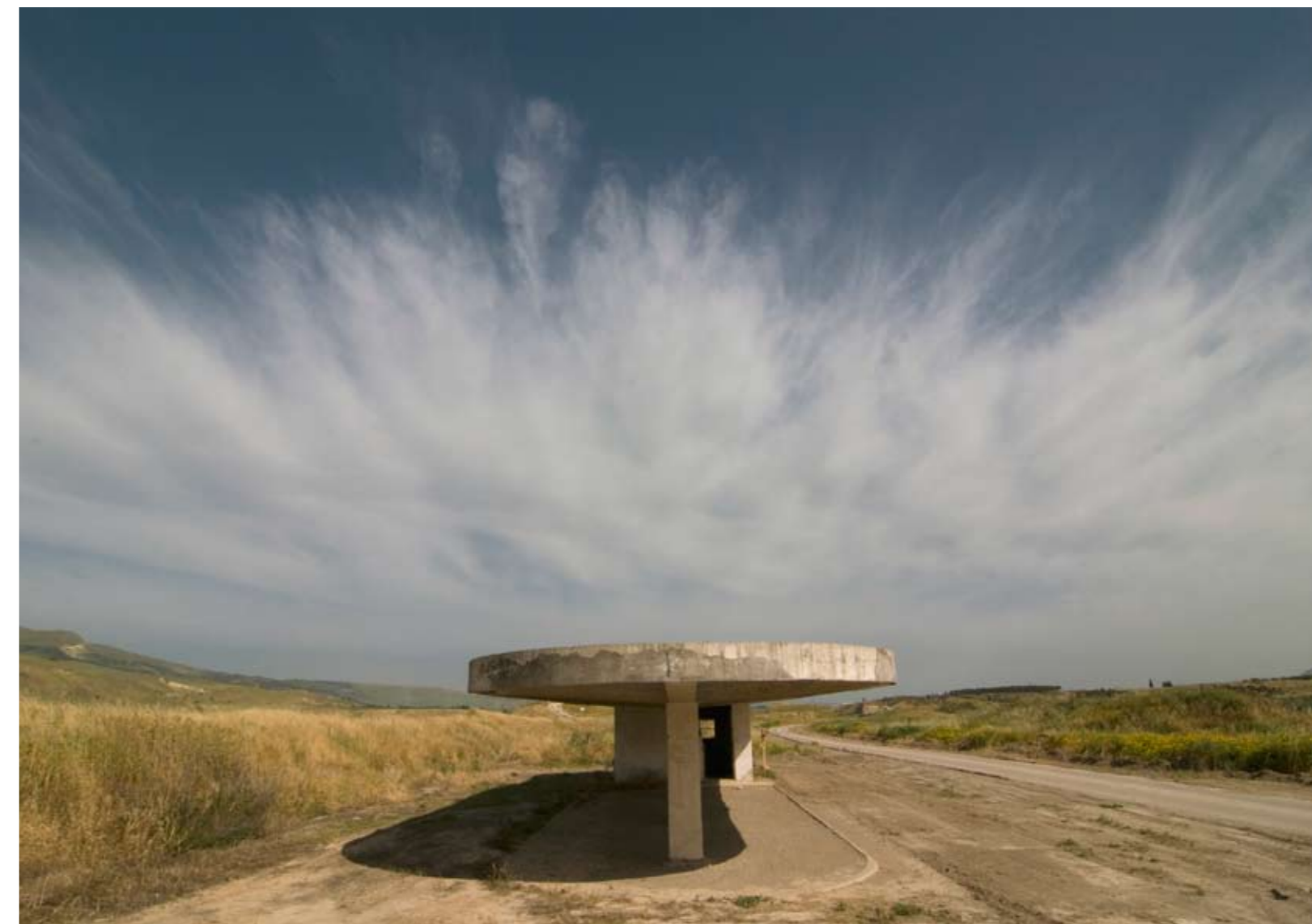
The Naharayim Train Station, inaugurated in 1932, enabled local residents and workers at the power plant to access Haifa or Damascus with ease.
