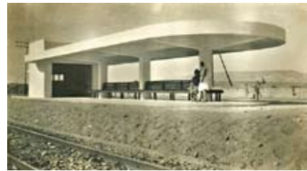
Naharayim Train Station on the Hejaz Railway, circa 1932.
