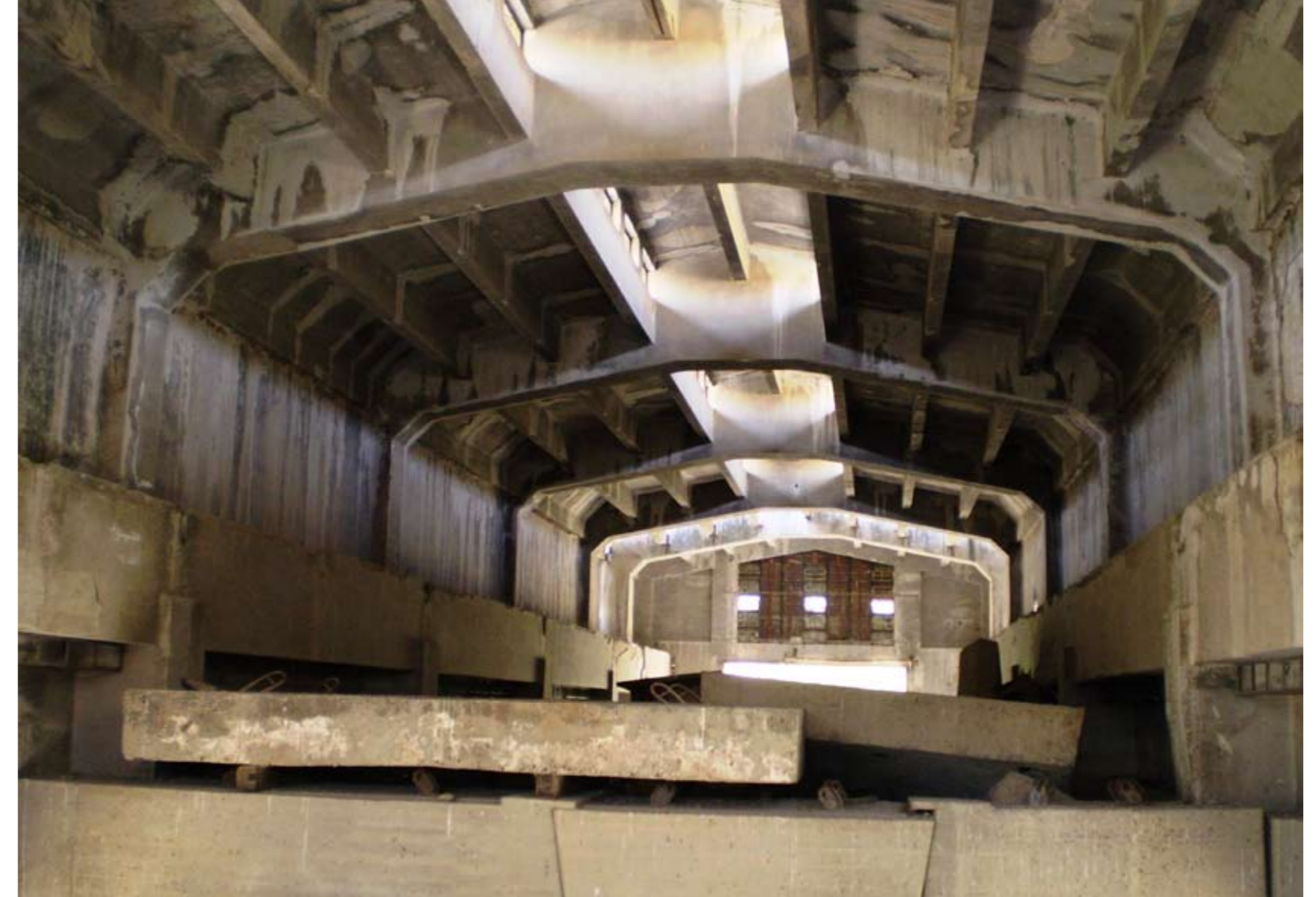
The former turbine building will be adapted for use as a visitor's center to tell the story of the shared cultural and natural heritage of the Jordan River Valley.
