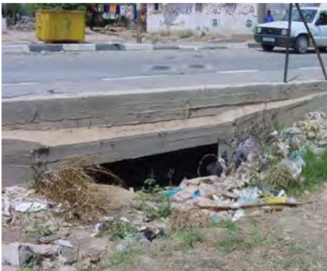
Figure 1: Current situation of drain pipes
