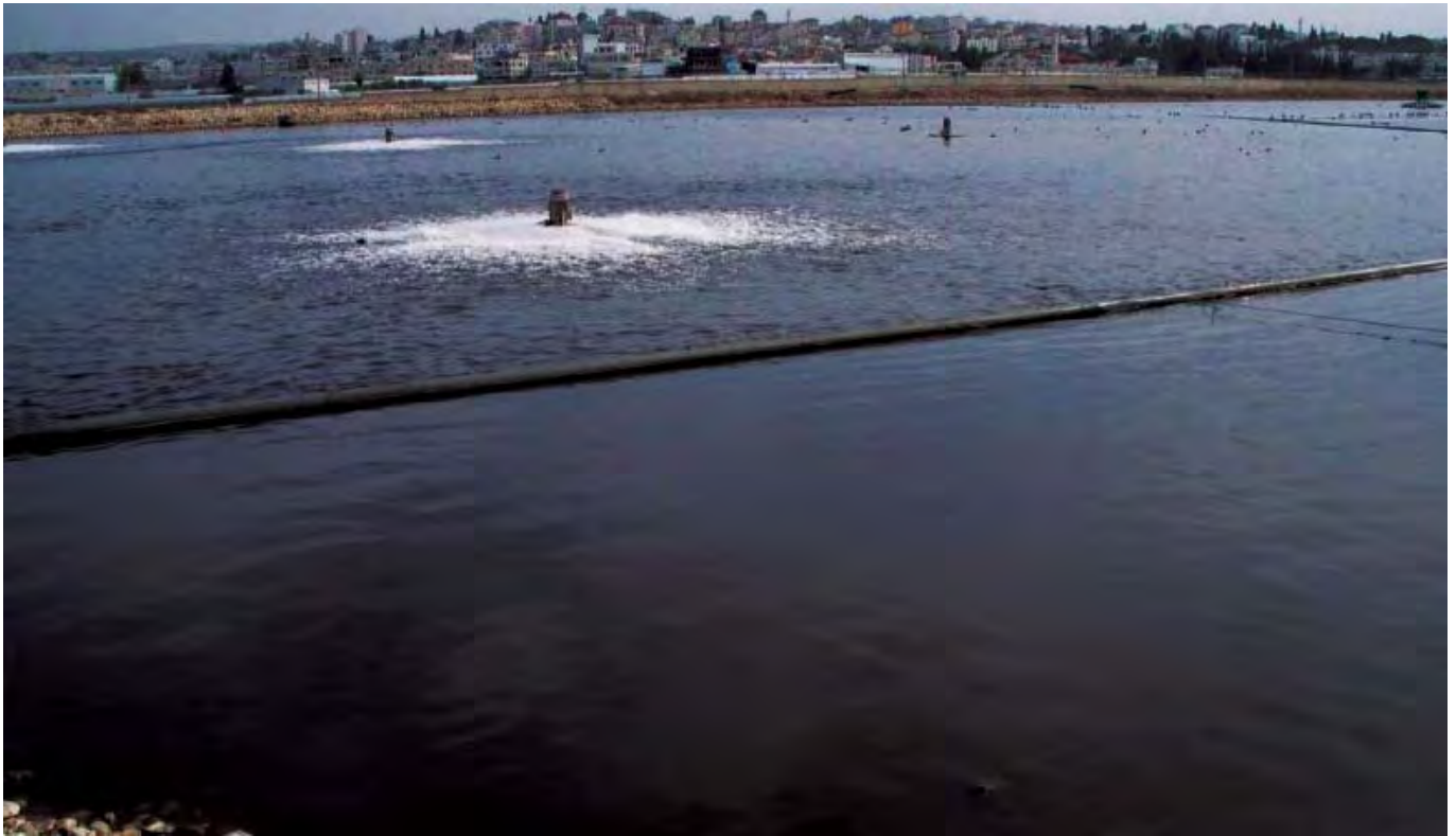
Figure 4: Aeration ponds at Yad Hana WWTP with the city of Tulkarem in the background. Source: Rehabilitation of Alexander Stream, DHV and Tsalul, April 2011.
