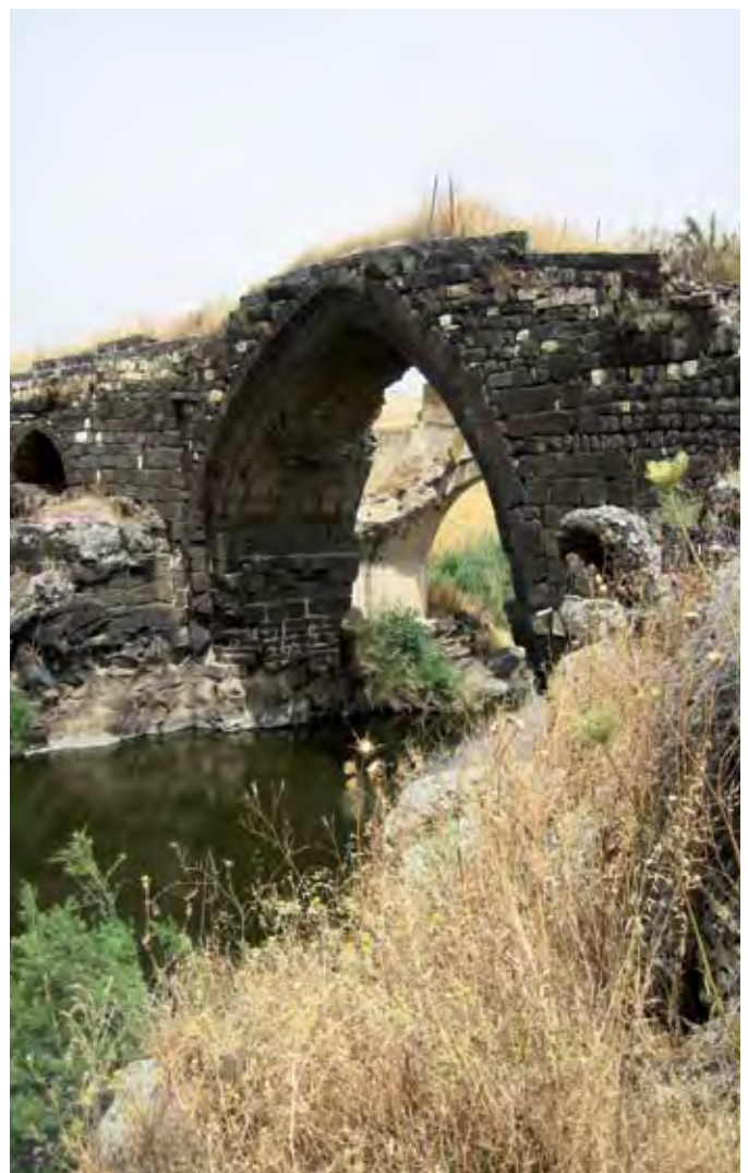
Figure 4: Roman bridge at Old Gesher/Jeser Al Majama, Photo: FoEME
