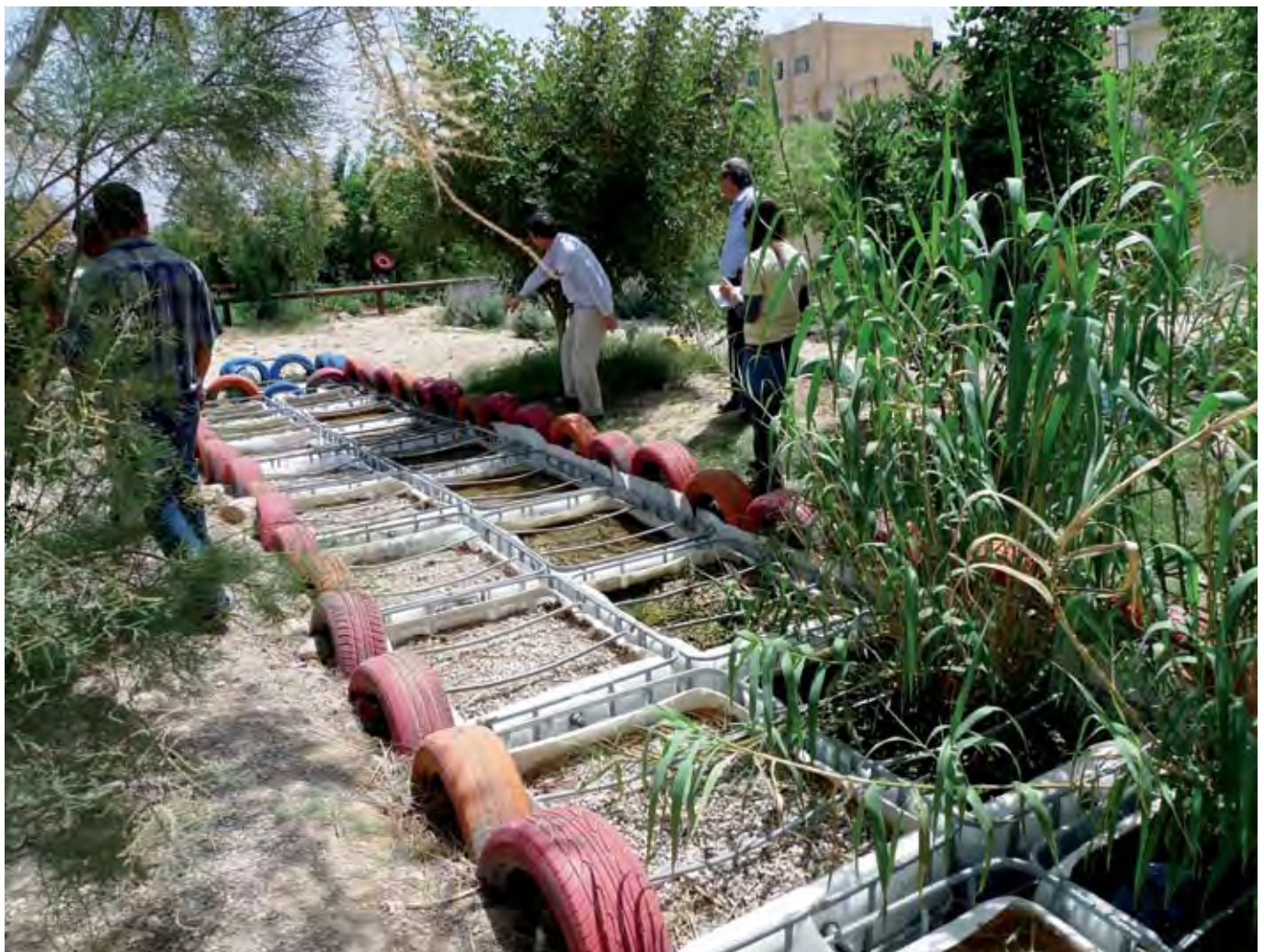
Figure 3: Ecological greywater treatment system at Auja Eco-Center, Photo: FoEME
