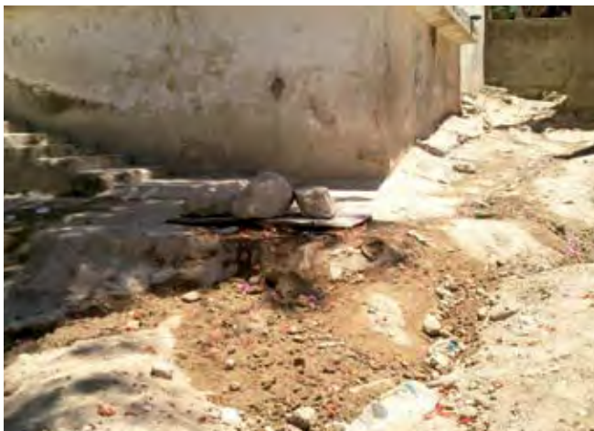
Figure 1: Poorly covered cesspit, June 2012, Photo: FoEME
