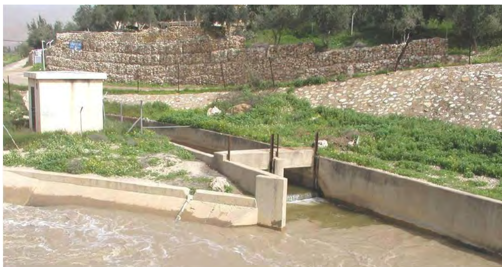
Figure 37 - Mixing of water from the KAC with water from the King Talal Dam
