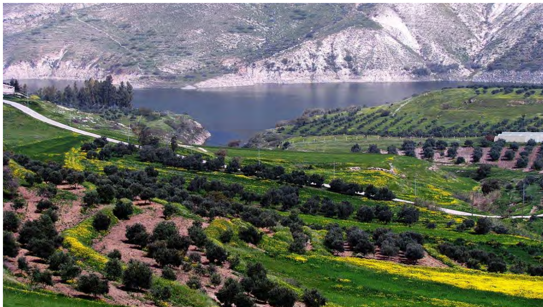
Figure 8 – The Arab Dam
