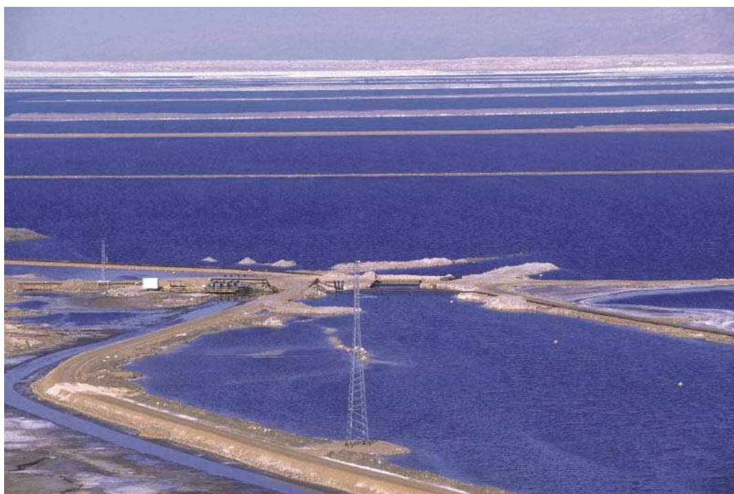
Israeli and Jordanian industries use evaporation for low-cost extraction of the Dead Sea's minerals
